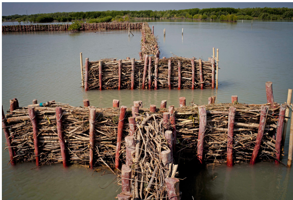
Figure 4a. An example of a permeable groin structure erected in 2013.
