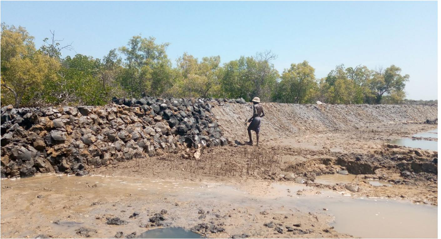
Plate 3.15. Salt pans are majorly constructed behind mangrove areas on bare salt flats. Operators claim that this is important because presence of intact mangroves in front of the salt pans ensure safety of the pans at times of rough and strong waves and tides that often break the dikes.
