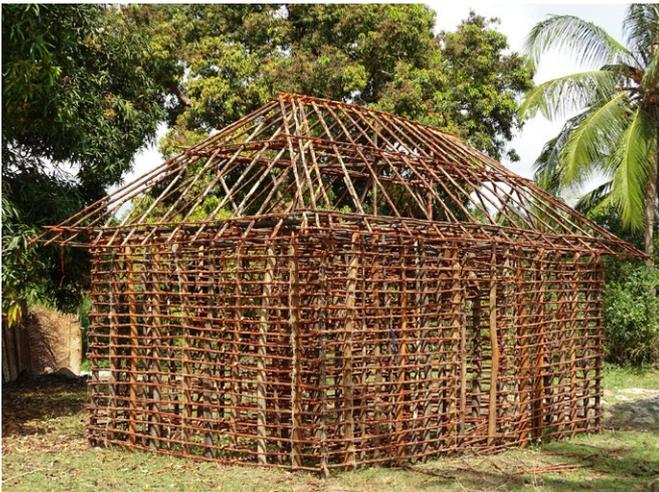
Plate 3.4. House construction by mangrove poles and timber, pasted with mud and roofed by corrugated iron sheets are common in mangrove areas, for example, these ones were found at Mfisini Village in Rufiji Delta.
