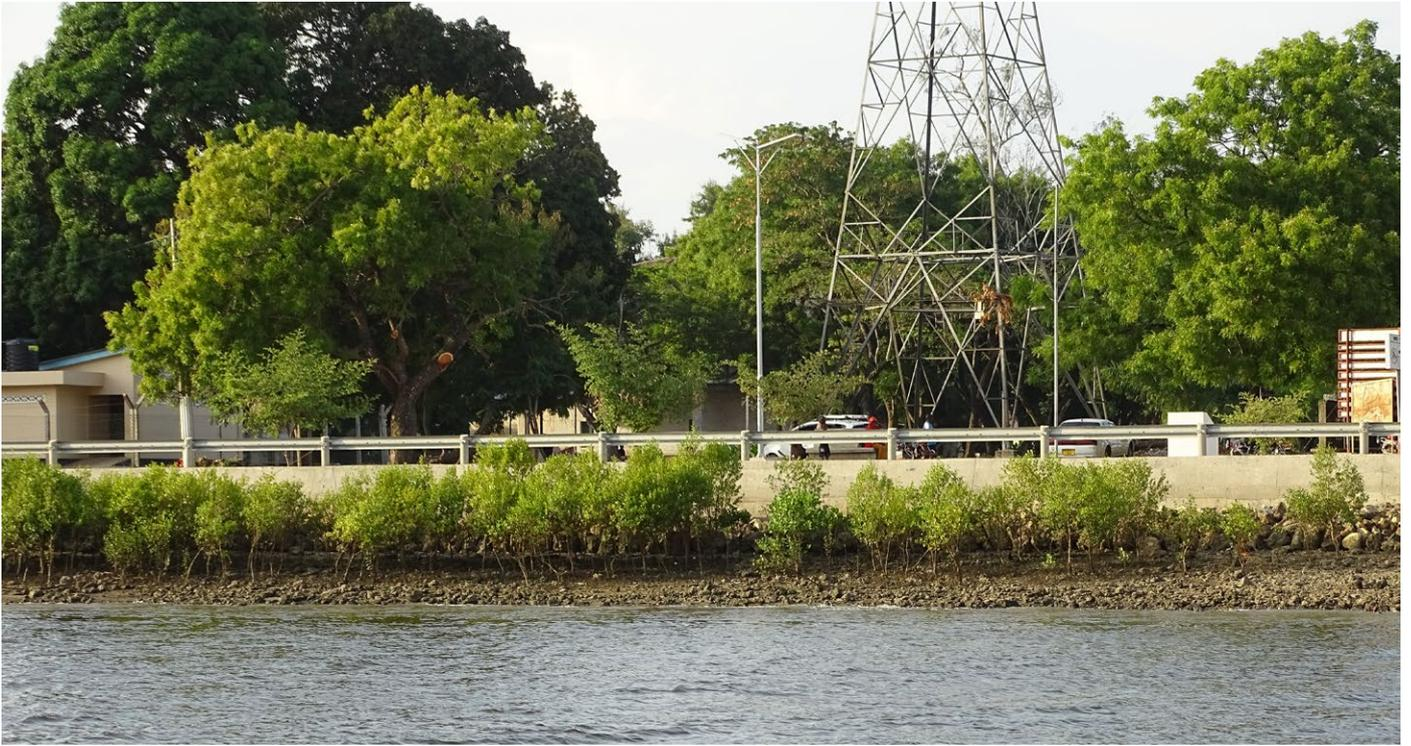
Plate 2.7. Constructed seawall and planted mangroves to protect it at Pangani Town for protection of settlements and properties from coastal/river bank erosion. The seawall has added another value of being a recreation area.
